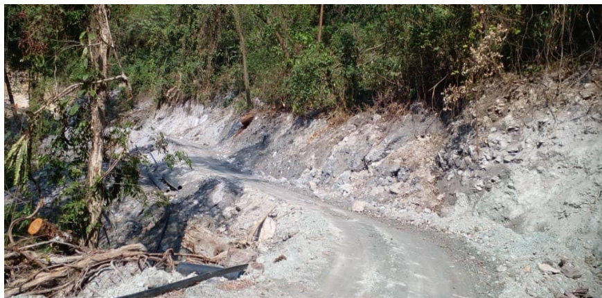
Figure 8. New Road for water Infrastructure
