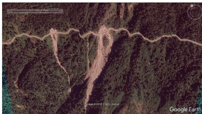
Figure 12: overview of debris dumped along Phuentsholing-Thimphu road
