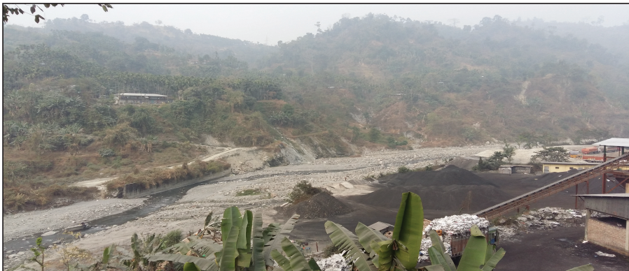
Figure 16: Photo showing waste dumped from factories along the river bank (right) and affected road to Phurbaling village(left)
