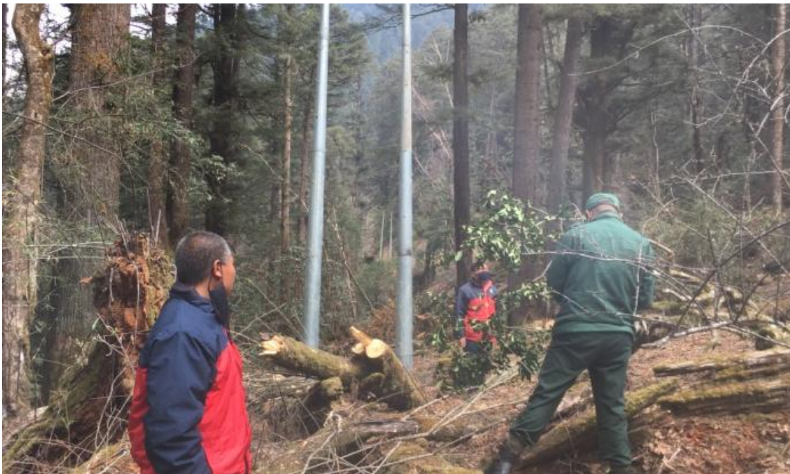
Figure 11: Felling of trees along electrical transmission line
