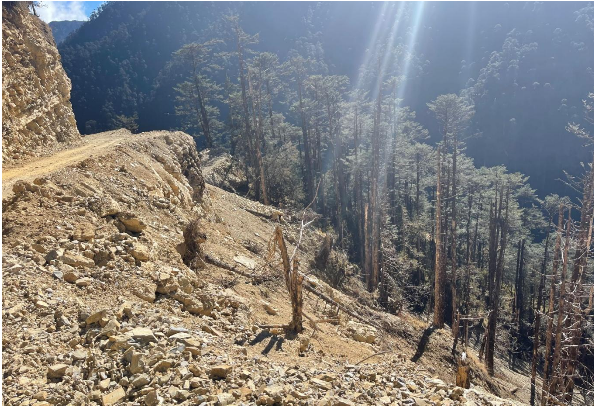
Figure 12: Deep excavation along Dodena-Barshong road
