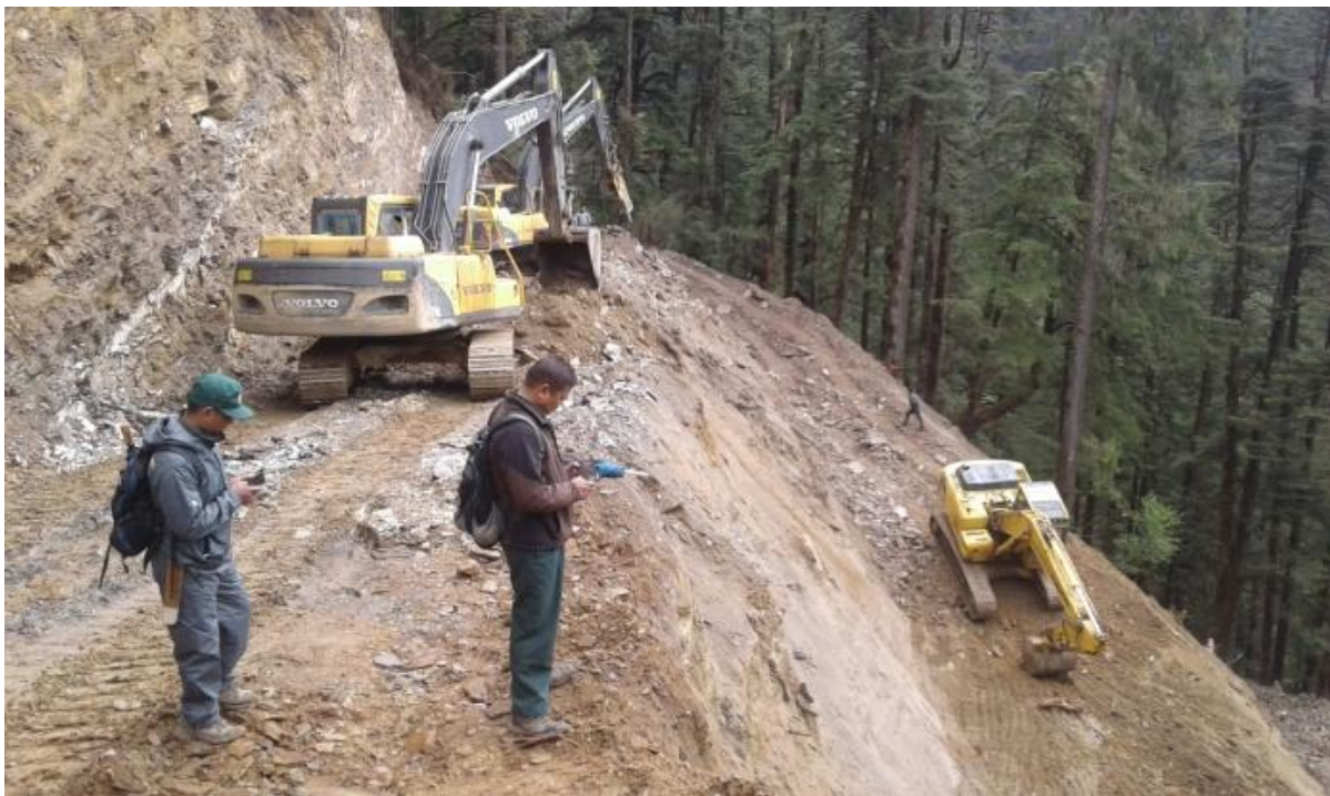
Figure 10: Construction of Barshong GC road
