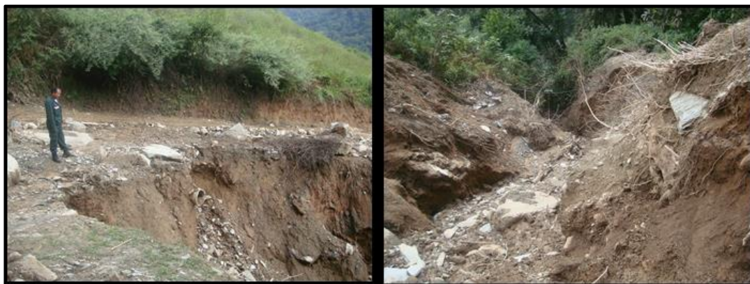
(A) Photo 3: Landslides within watershed (B)
