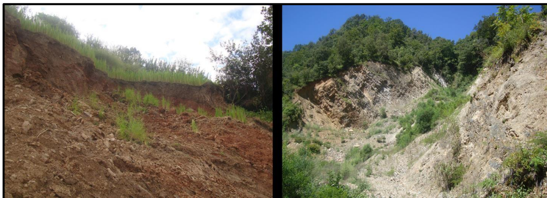
Photo 10: Landslides in watershed
