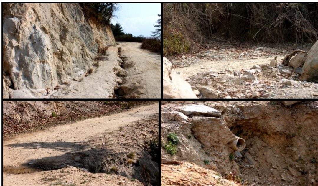
Photo 1: (A) Absence of drainage on farm roads & water channel formation. (B) Lack of catch pits on depressions & streams along farm roads. (C) Blockage of hum pipes being too small in size & also due to lack of catch pits and debris entering & blocking the hume pipe diverting water onto farm roads. (D) Gully formation on farm roads
