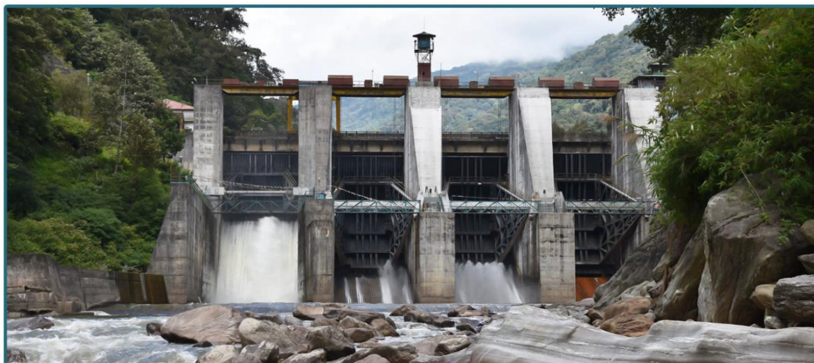
Figure 2.3: Appurtenant Structures include spillway gates and gate lifting equipment
