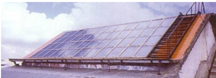
Figure: 4.16: Solar Air Heating System used in Cold Climate
