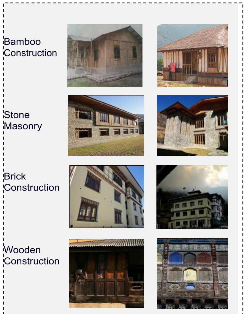
Figure 2.6: Use of materials for wall construction in Bhutan
