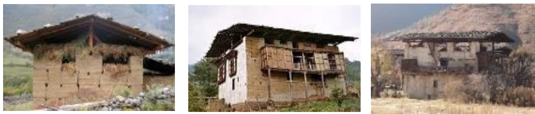
Figure 2.4: Typical rammed earth buildings in Bhutan
