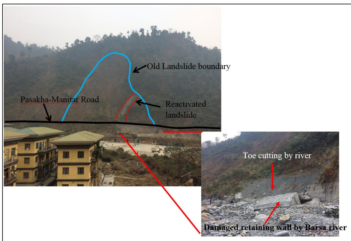
Figure 14. Landslide (Inventory ID: lsd02150230) seen from the BFAL colony.
