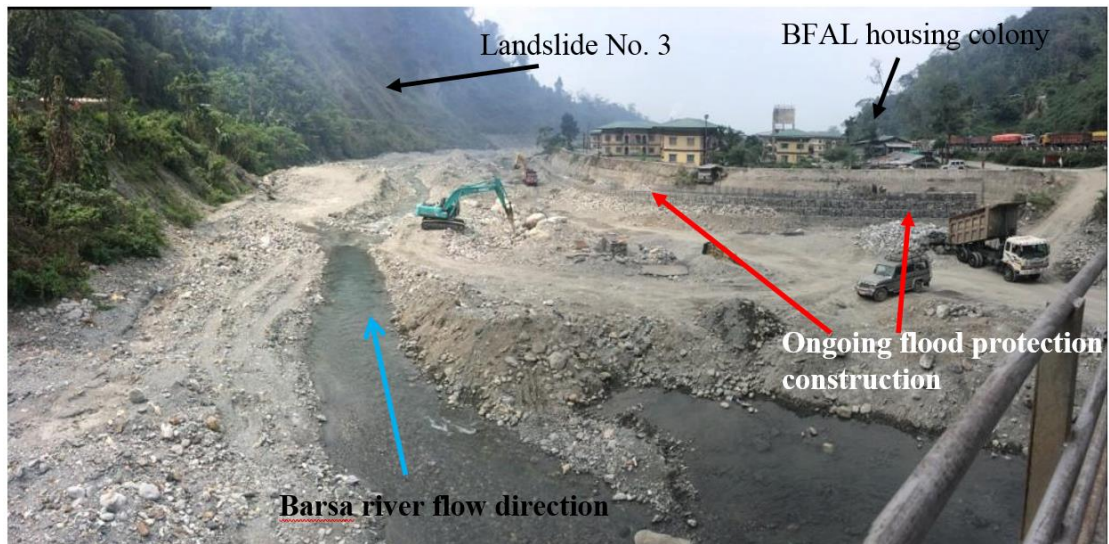
Figure 15. Disturbance in Barsa river course due to ongoing river protection wall.
