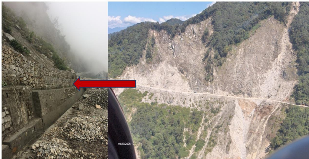
Figure 12. Jumja slide with bulging retaining wall as shown in the picture. Inventory ID: Isd02100141 .
