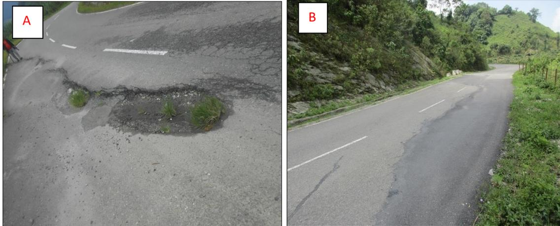
Figure 12. A) The sight of the road at Arong with a clear crack on August 2015. B) The same sight of the road after blacktopping on May 2017.
