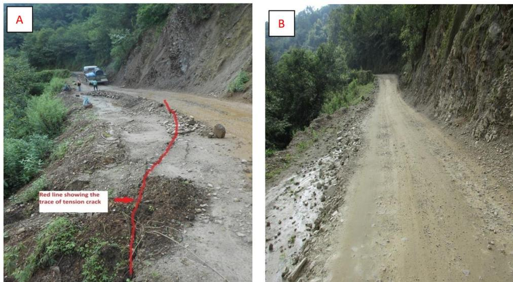
Figure 13. A) The sight of the road at Moshi with a red line showing the crack on August 2015. B) The same sight of the road after filling up with rock and soil on May 2017 without clear sight of tension crack.
