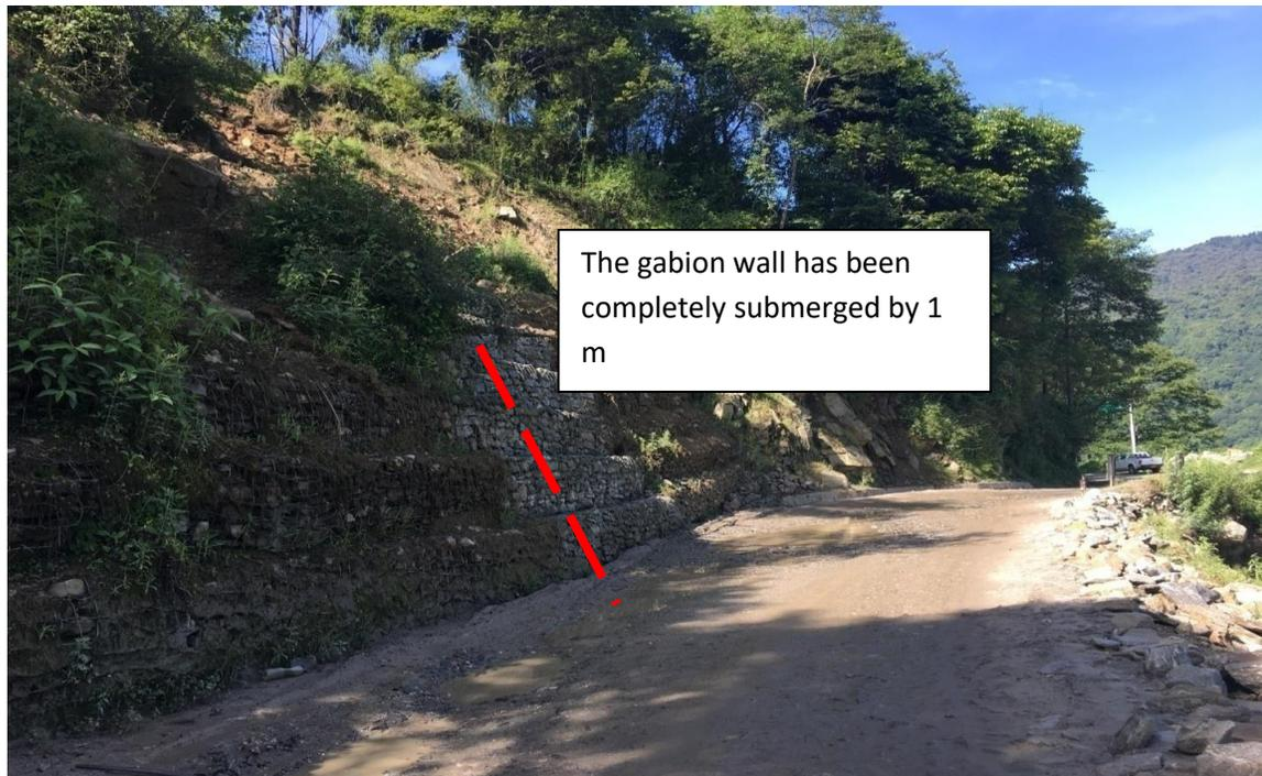
Figure 11. Gabion wall has completely submerged by 1 m at Tsimasham landslide. Refer Figure 10 for comparison (Picture taken in May 2017).
