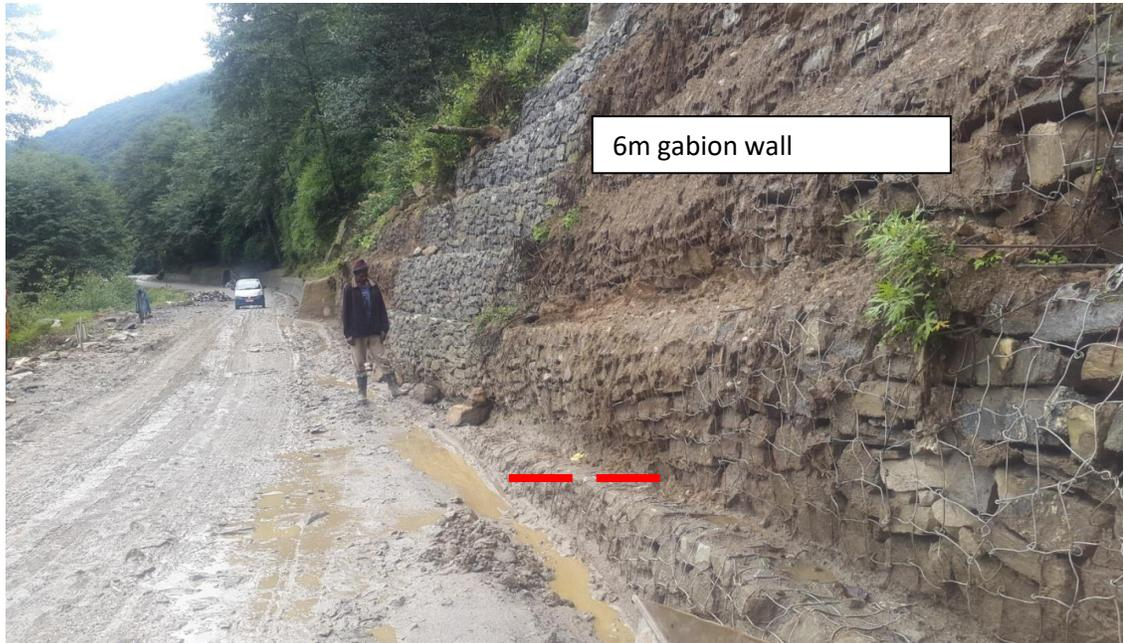
Figure 10. The sinking of Gabion wall indicating active mass movement at Tsimasham landslide (Picture taken in September 2016)
