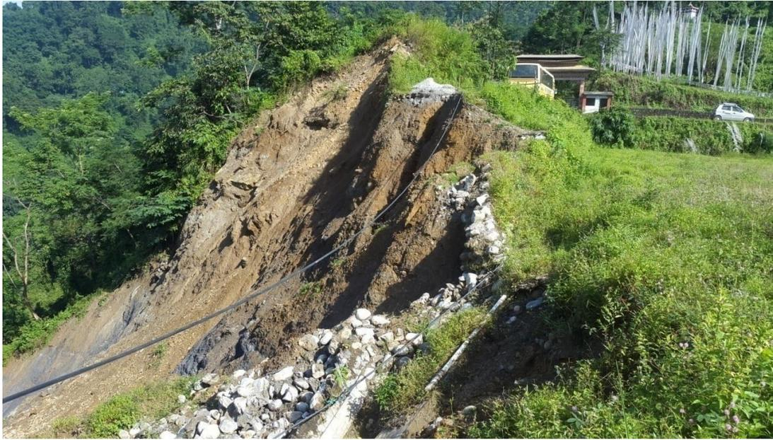
*Figure 12. Tension crack completely washed away at Reldri (Picture taken in May 2016).*
