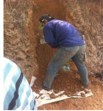
Figure 5. Materials observed in the pit no.3.
